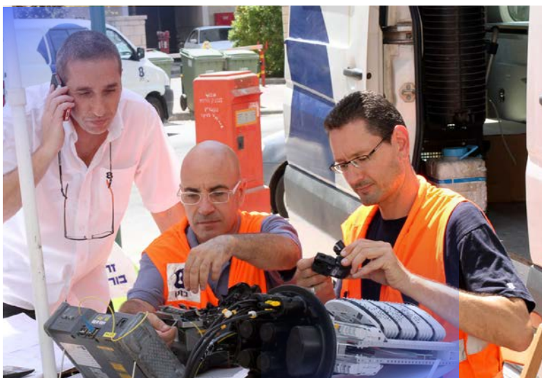
Bezeq technicians installing fiber
